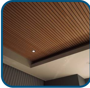
● Aluminum Suspended Ceiling
